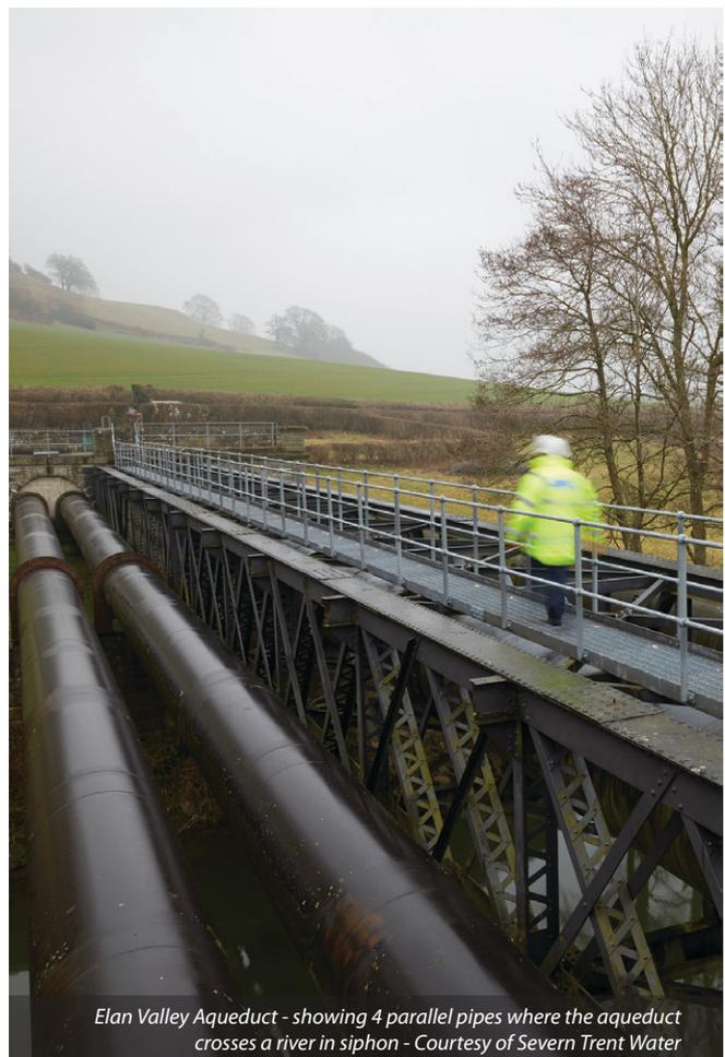
Elan Valley Aqueduct - showing 4 parallel pipes where the aqueduct crosses a river in siphon - Courtesy of Severn Trent Water
