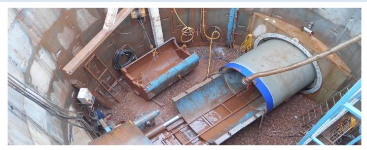
The new sewer was required to connect with the existing Wessex Water sewerage network at fixed invert levels and also cross beneath a number of services and features which cannot be diverted or avoided, and therefore constrain the levels and gradients at which the sewer can be constructed.
